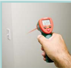
Check building for insufficient insulation
